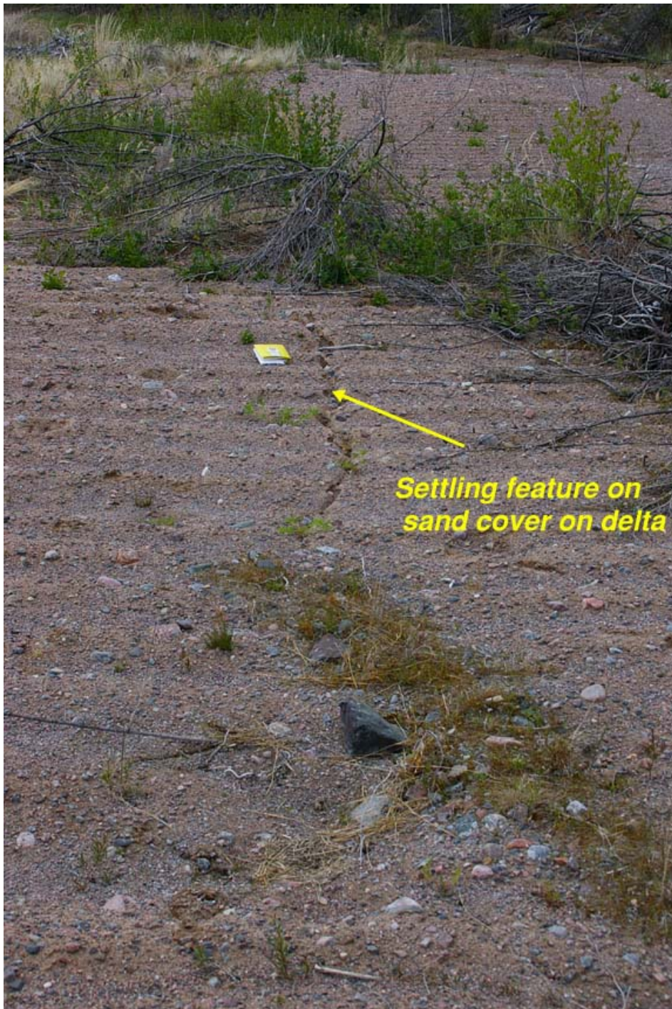
Photo 13 – Settling feature in sand cover at Fookes Delta (location corresponds with “Settling on Delta #2” of Photo10)
