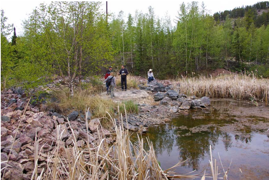
Photo 4 – Marie Reservoir at outlet (note: water significantly below flow point to spillway)
