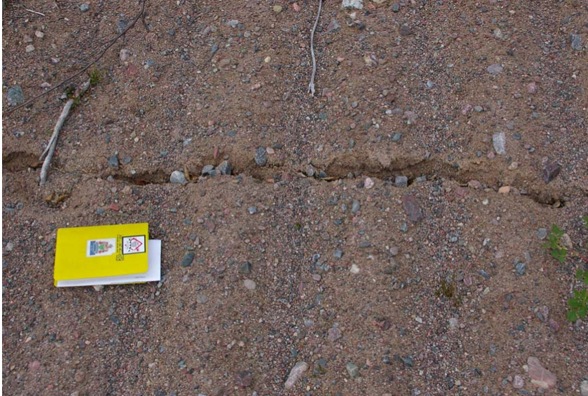
Photo 14 – Close-up of settling feature from previous photo
