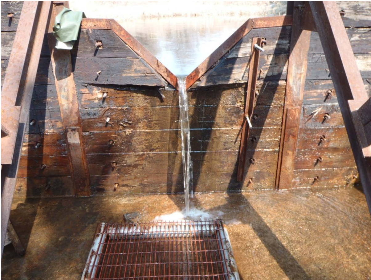
Figure 4: Photograph of Damaged V-notch Weir at Fulton Creek (TL-7)
