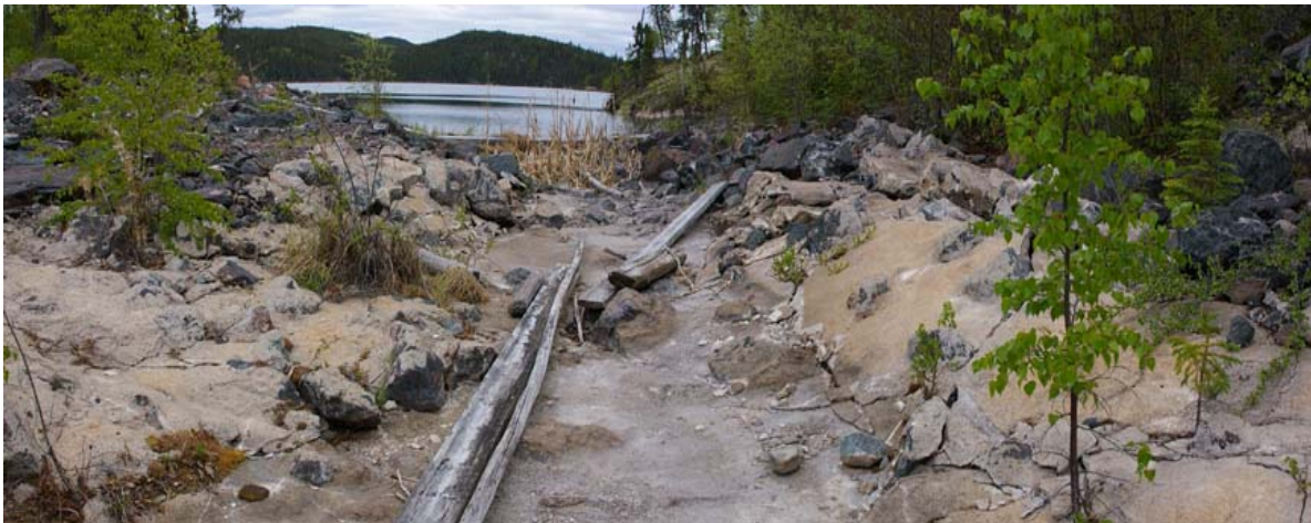
Photo 5 – Fookes Reservoir Spillway looking upstream (no flow in spillway)
