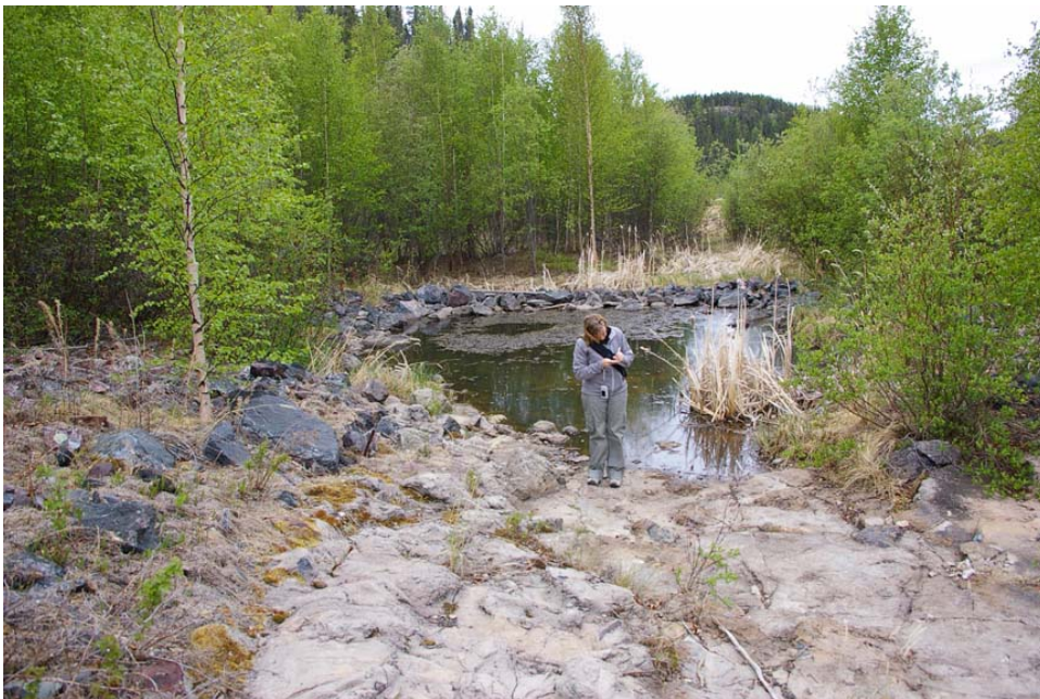
Photo 2 – Marie Reservoir Spillway looking downstream to stagnant stilling basin
