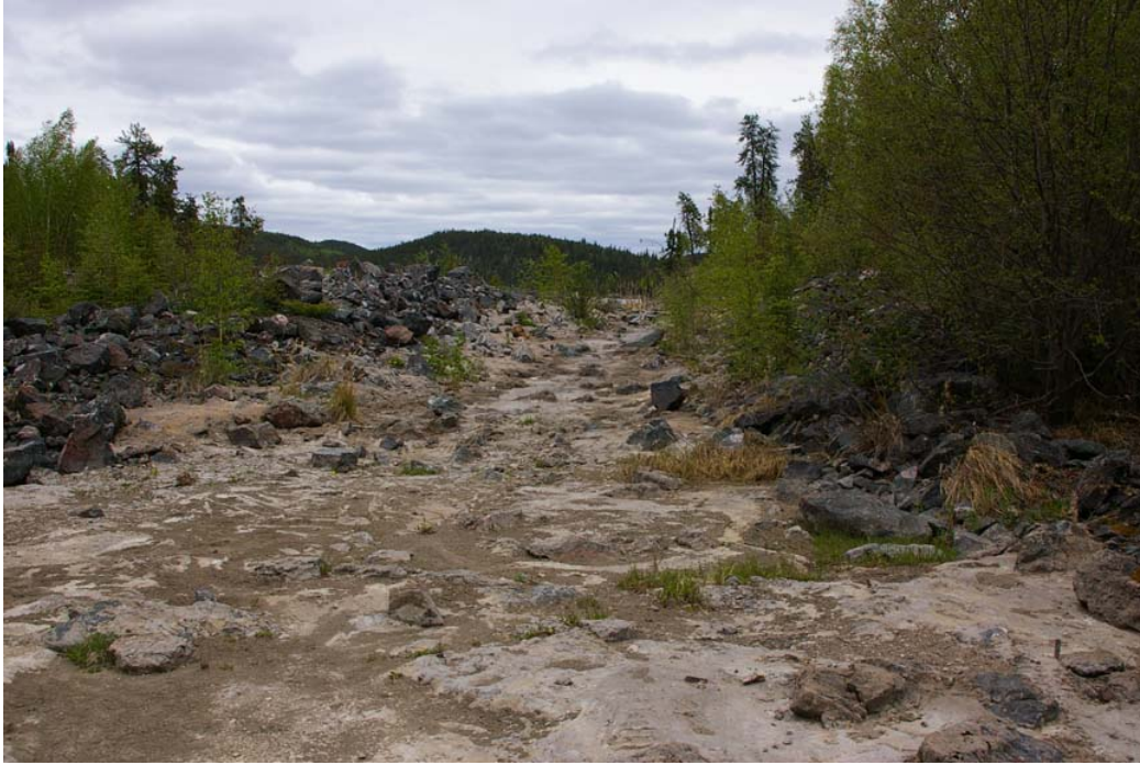
Photo 6 – Fookes Reservoir Spillway looking upstream from stilling basin
