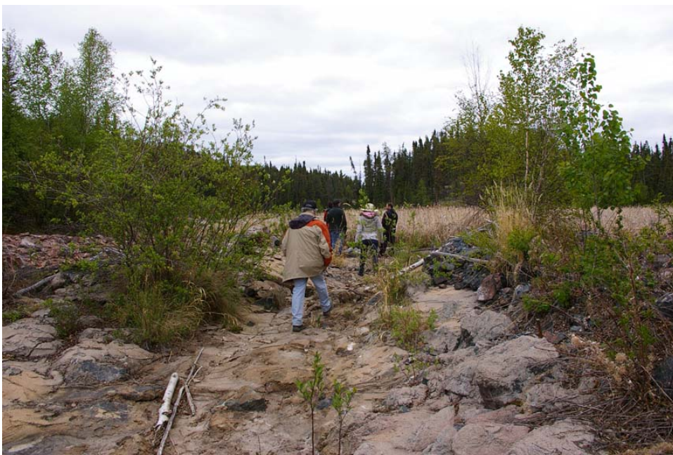
Photo 1 – Marie Reservoir Spillway looking upstream (no flow in spillway)
