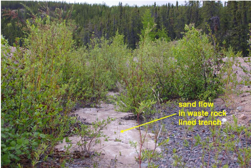
Photo 11 – Sand flow feature in trench lined with waste rock
