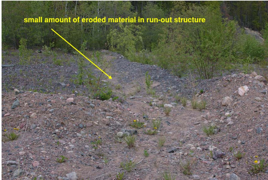
Photo 16 – Run-out structure along north access road
